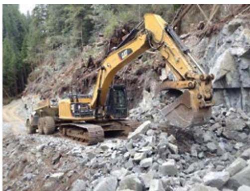
The slide occurred as the operator was entering an end haul transition zone in moderately steep ground in an area containing subsurface water and deep, wet organics not identified in the construction plan.
