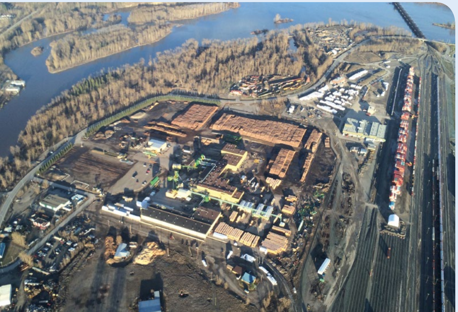
TOP: Aerial shot of Lakeland Mills. The green pipe bridge supports the piping for the DDES before it heads under the rail track to downtown Prince George (which is off the right side of the photo).
