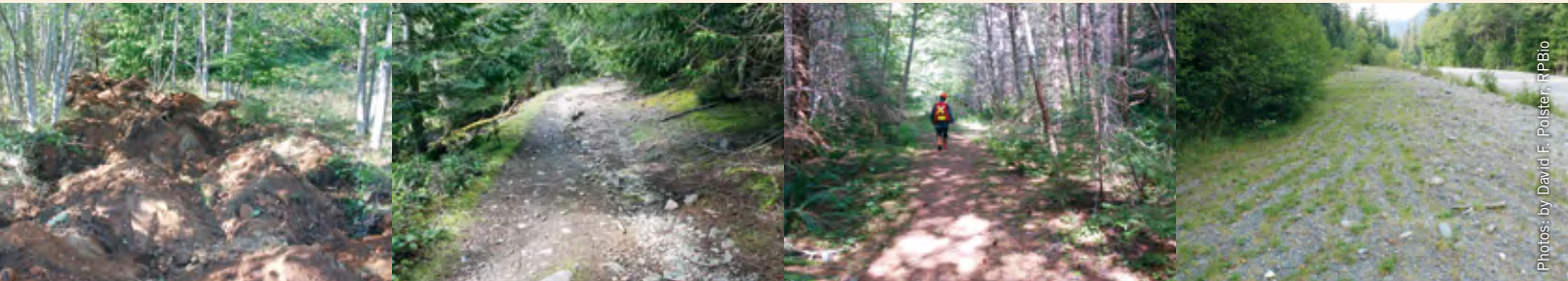
Captions from LEFT: A) The rough and loose treatment on this old forest road will solve a number of issues and allow natural processes to restore the road. B) Compacted old road surfaces intercept near-surface groundwater and promote erosion. C) Compacted road surfaces prevent the establishment of pioneering species that would initiate the natural recovery processes. D) This road surface was scratched with the teeth of an excavator bucket resulting in a few cm. of de-compaction; not enough to allow forest growth.
