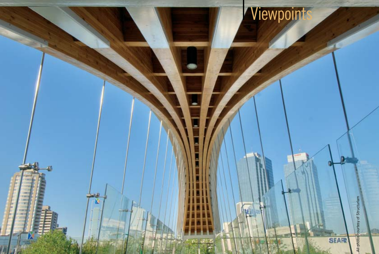
These 130 ft glulam arches made from Douglas-fir span Kingsway in Burnaby and support a pedestrian walkway.
