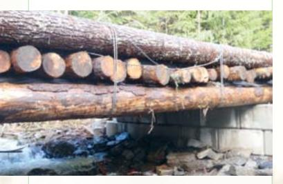
RECENT LOG STRINGER BRIDGE FAILURES HAVE RESULTED IN AN increased awareness of the complexities involved in the design, construction, and assurance of these structures. More specifically, the load effects produced by tracked vehicles when travelling over these structures without the use of lowbed equipment has become a concern especially as the shift is made to smaller diameter stands such as lodgepole pine or second growth Douglas-fir.
