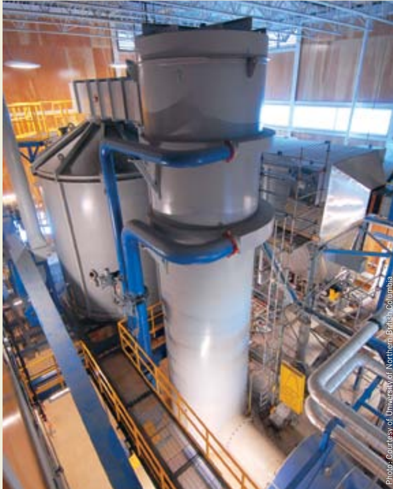
Innovations like the wood gasification power plant at UNBC and the associated research is a good example of how things could change.
