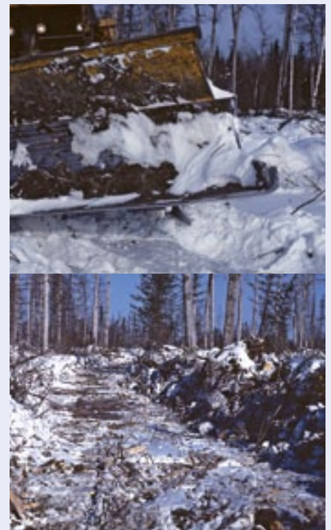
Figure 2 A & B. Crawler tractor with a Rome KG blade used for stump shearing. An in-block winter access road built using stump shearing.
