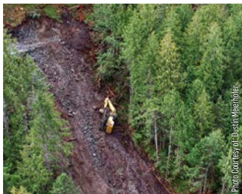
Significant construction initiated slide event on BC's coast involving road construction on a moderate to moderately steep slope through a wet draw containing organics over compact sandy-clay soils.
